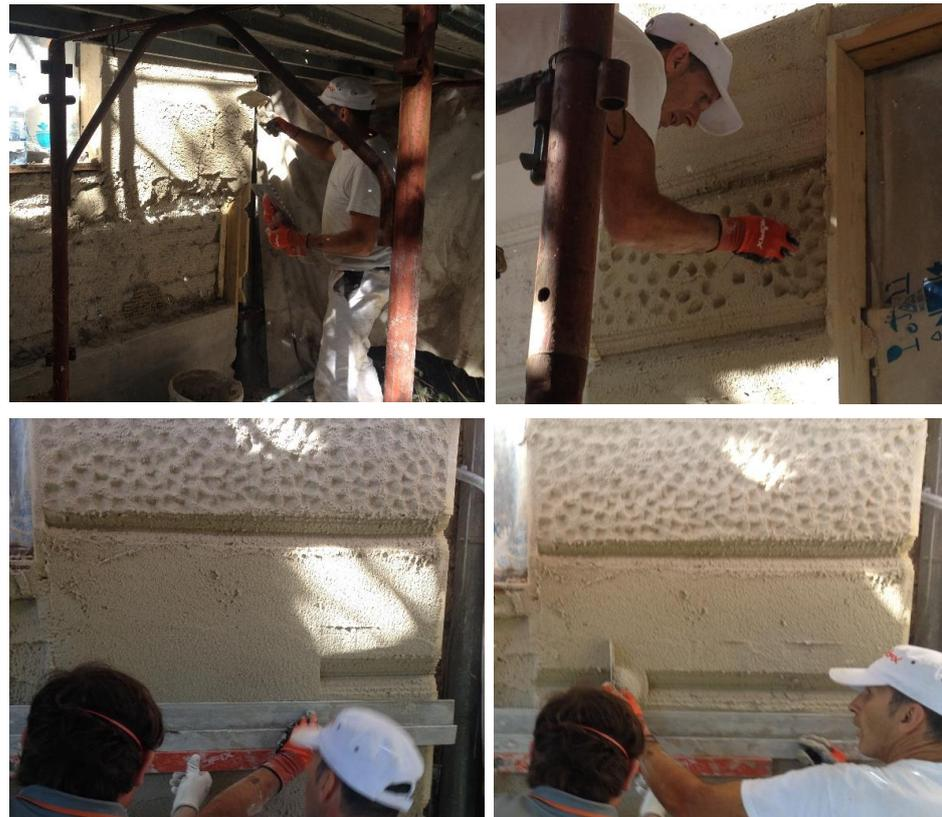
**Figure 3.** Stepwise application of the aerogel-based rendering without reinforcement mesh to an external façade, and processing to mimic decorative elements of the original façade. A clear indication for its advantageous high workability.
